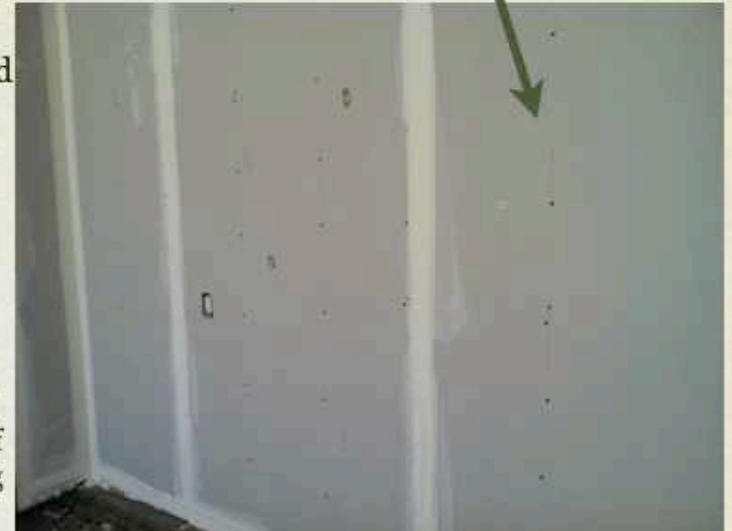
Gypsum Wallboard: June 1, 2013 SS Builders
