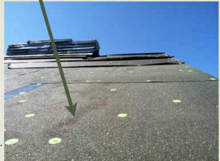
Asphalt Coated Felt: June 1, 2013 SS Builders
