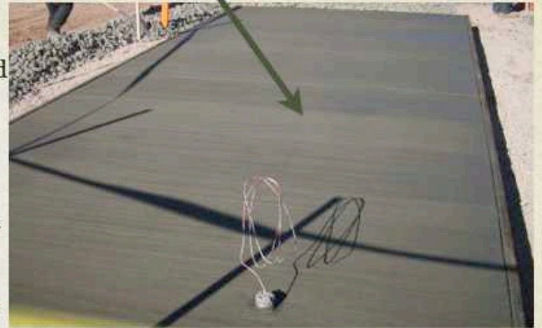
Concrete Paving: June 1, 2013 SS Builders
