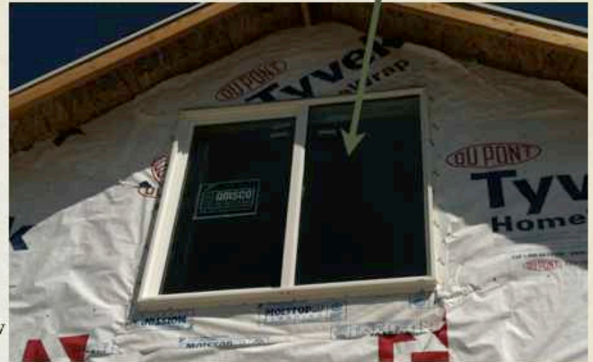
PVC Window: June 1, 2013 SS Builders
