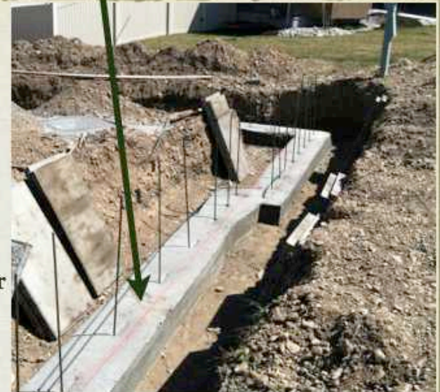
Footing: June 1, 2013 SS Builders
