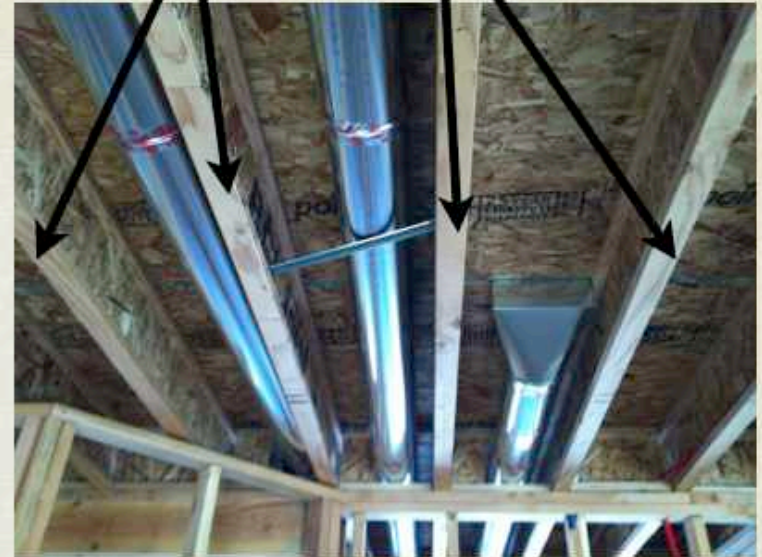
I Joist: June 1, 2013 SS Builders
