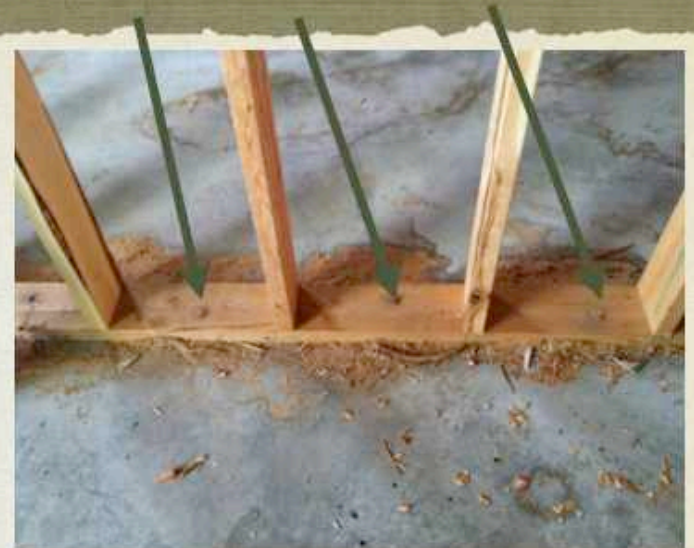
Anchor Bolts: June 1, 2013 SS Builders
