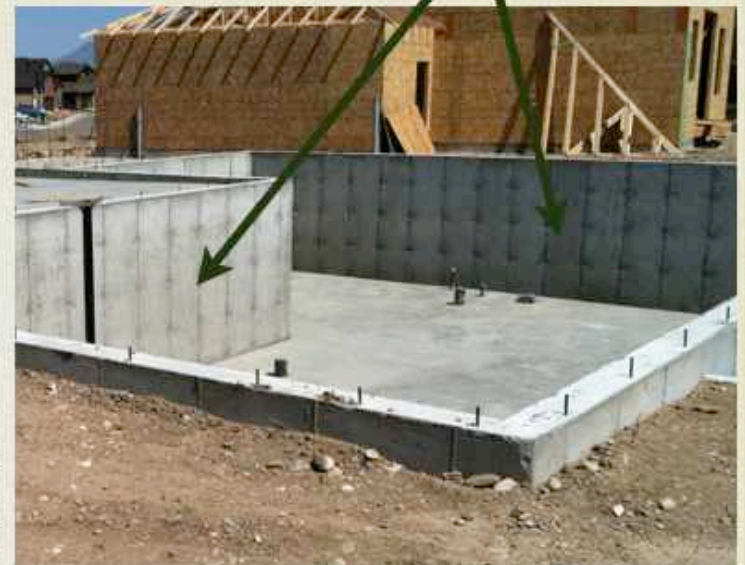
Concrete Wall: June 1, 2013 SS Builders
